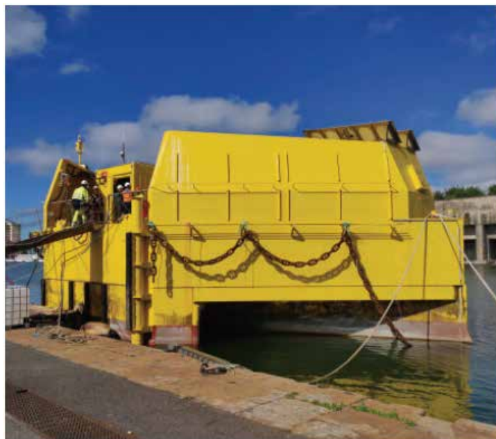
The production module, secured to a Wavegem wave energy structure, has been producing up to 400 kg/d of hydrogen since last September. COURTESY LHYFE
